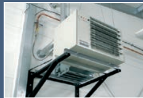
Horizontal installation of Monzun-RTI on the wall
