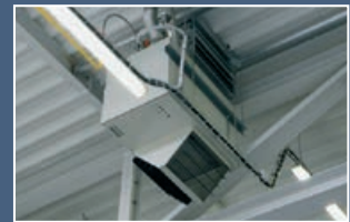
Vertical installation of Monzun RTI from the ceiling
